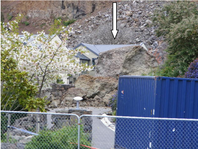
Rock in the driveway hard to move
