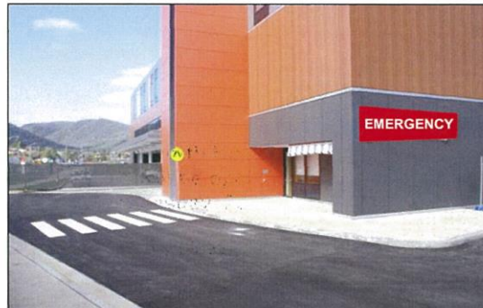
The new emergency department entrance and drop-off bay.
