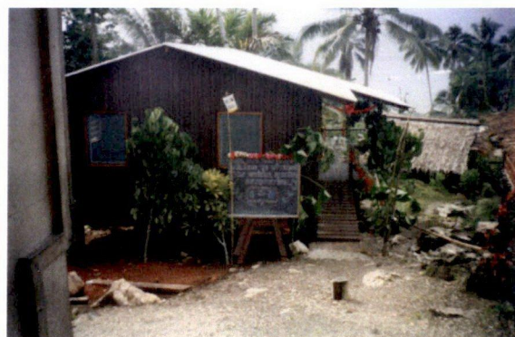
The project – a three bedroom maternity unit
